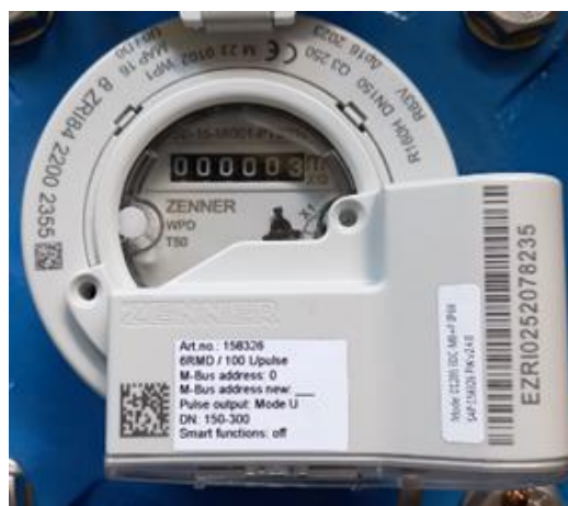
Figure 5: EDC mounting position
